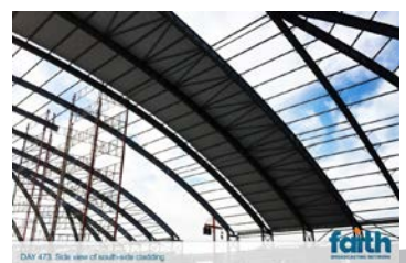
DAY 473: Side view of south-side cladding
