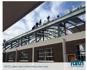
DAY 472: Insulation rolled out before cladding is fixed in place
