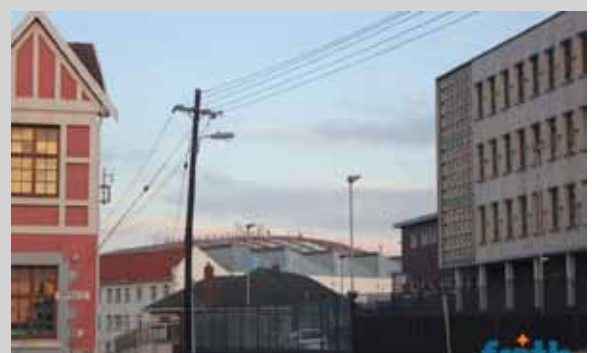
DAY 442: The dome construction peeking through the buildings
