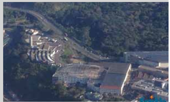
DAY 442: Aerial view of construction
